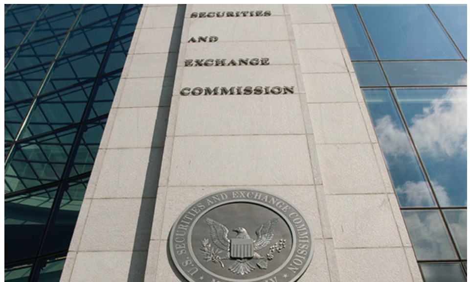
U.S. SECURITIES AND EXCHANGE COMMISSION BUILDING IN WASHINGTON.
